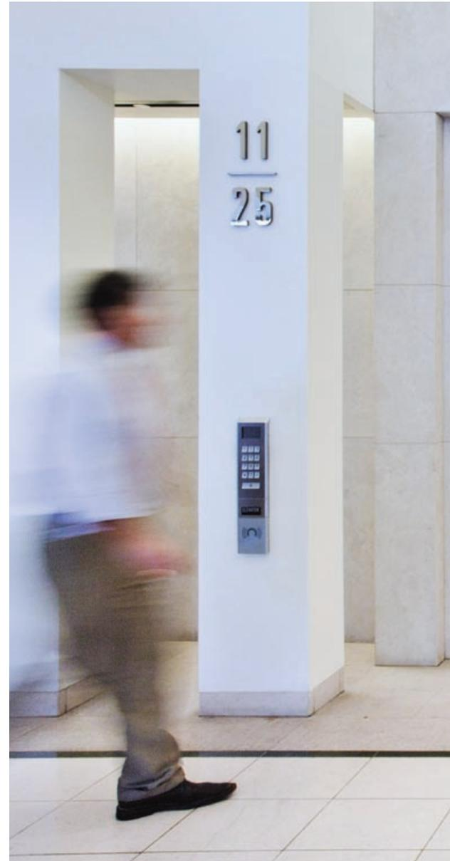
Schindler ID’s access control features validate passengers’ access rights and call an elevator automatically.
