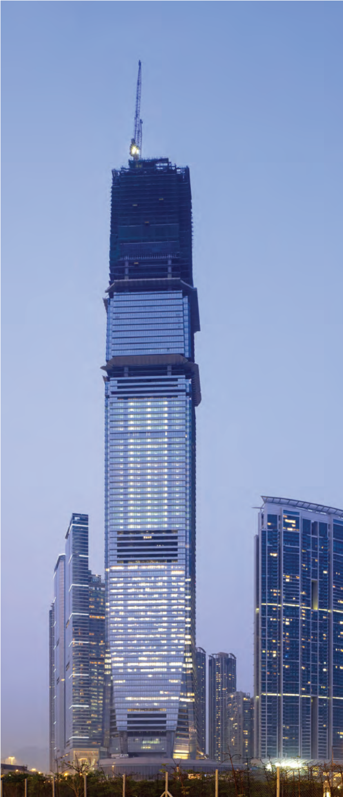
Figure 3: The tower under construction
